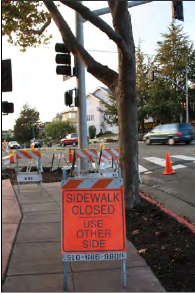
New signal installation, Rose and Grand
