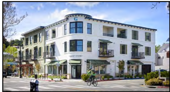
G Square Living is a market-rate, mixed-use development in San Rafael, CA. It has 10 units with a density of 59 dwelling units per acre.
