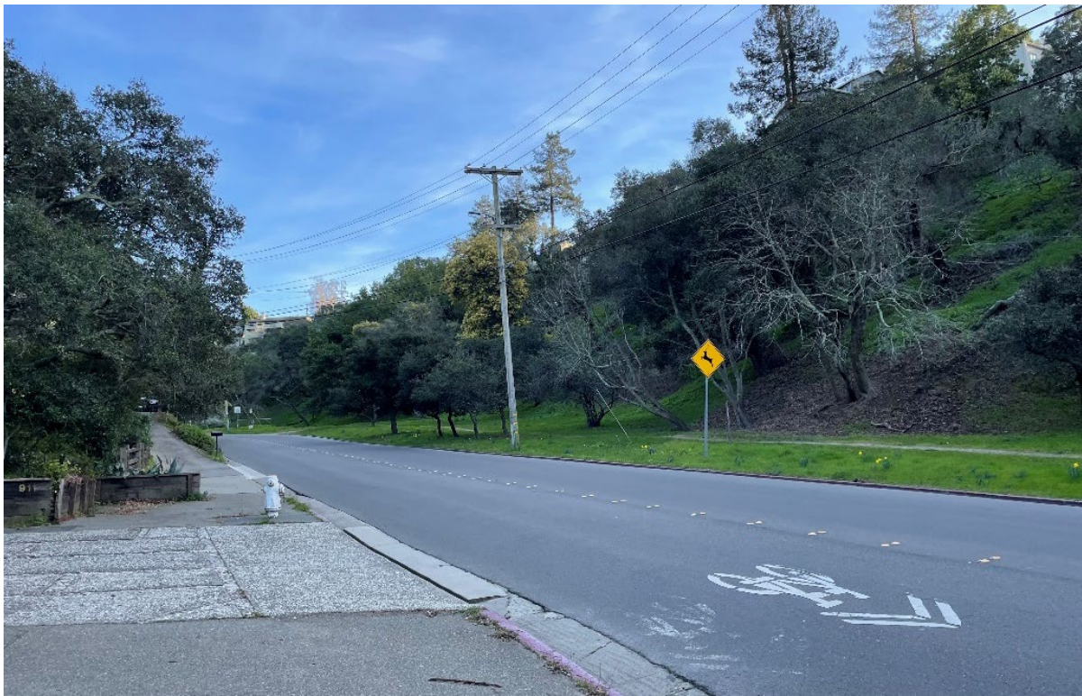
Photograph 3. View from intersection of Moraga Avenue and Red Rock Road looking southeast up Moraga Avenue towards Blair Park.
